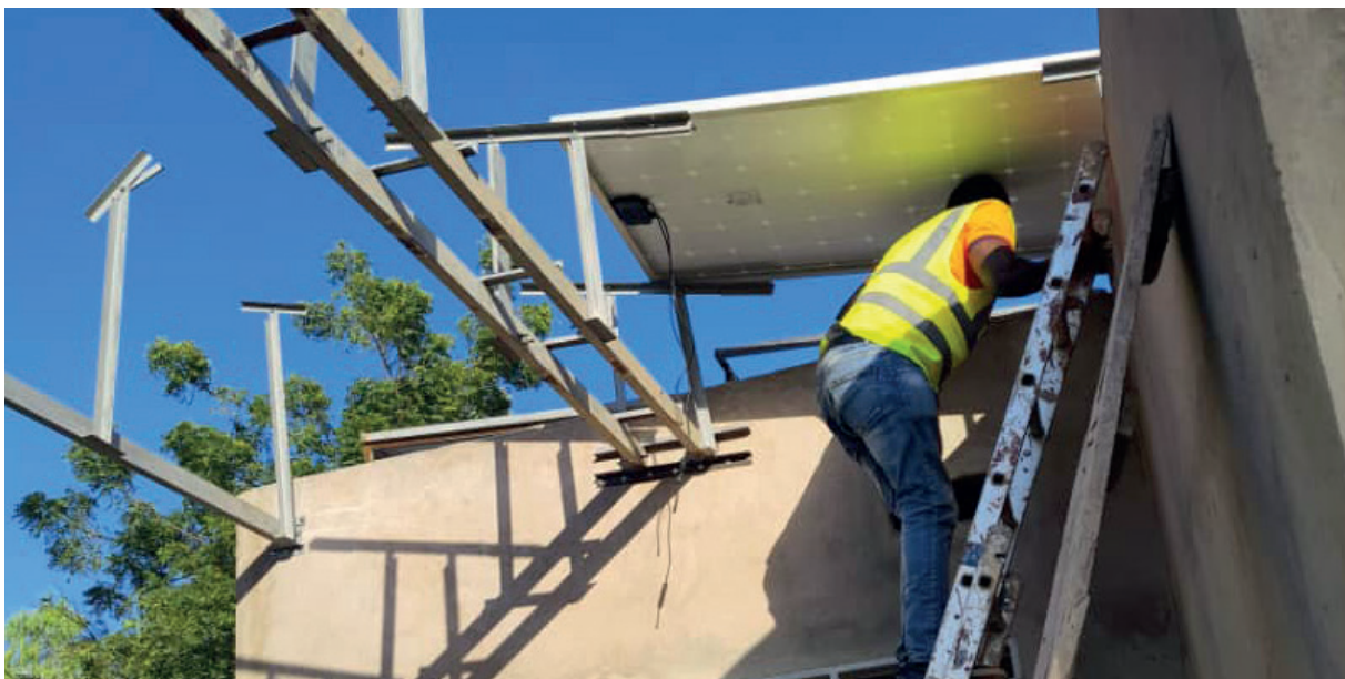
Installation of solar panels at the Clinic Wolobougou, near Bobo-Dioulasso, in Burkina Faso.
