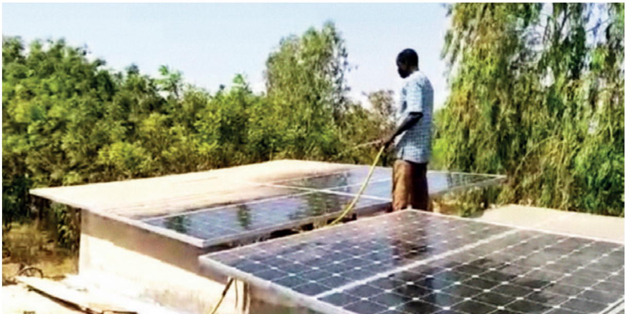
Solar system maintenance at the Clinic Wolobougou, near Bobo-Dioulasso, in Burkina Faso.
